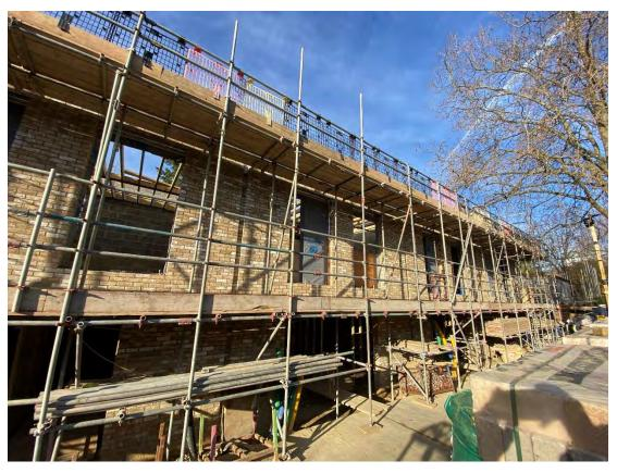
Mews Houses – Roof structure installed, ready for timber mansard structure to rear of Mews houses
