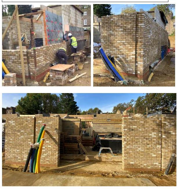
Mews Houses – Timber wall to rear of houses with Structural Steel running above Mews Houses – Structural Steel installed, with timber infills ready to receive First Floor joists
