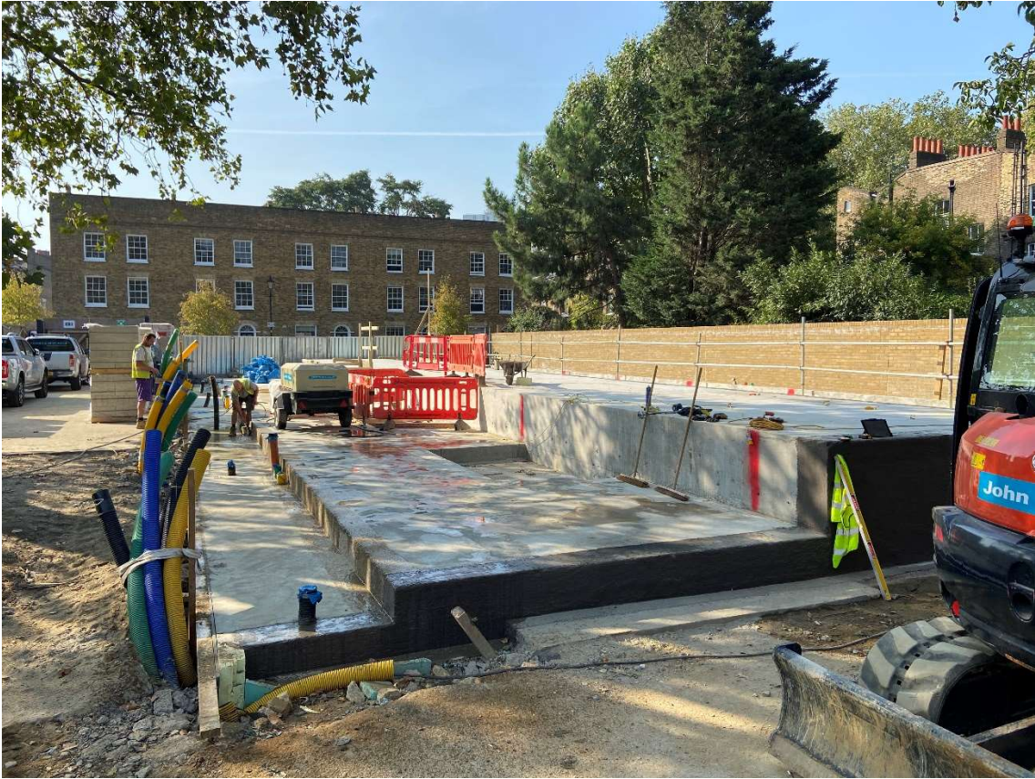
Mews Houses – Ground Floor Slab, structural waterproofing underway Mews House – Drainage to rear gardens
